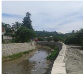
Figure 4. The flooded area where the embankment has been built
