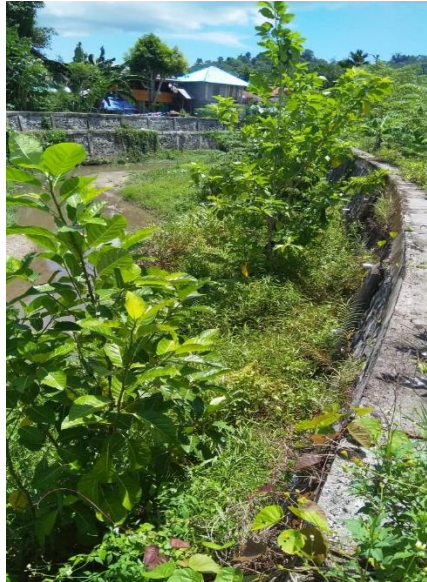
Figure 4 The flooded area where the embankment has been built
