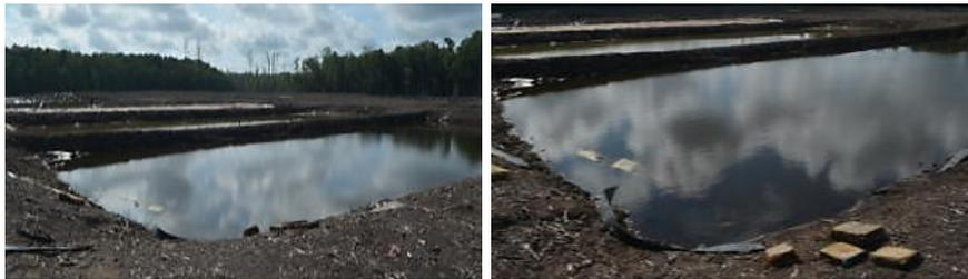
Gambar 4.3. Bak Water Treatment (Sediment Pond)
