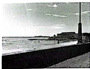
Sea wall built to protect the coast
