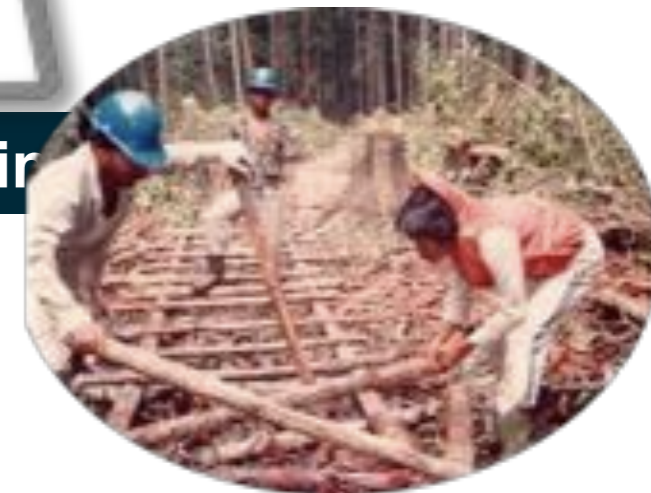
Skidding track construction
