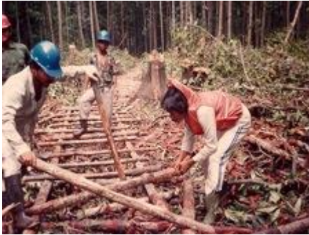
Figure 2. Skidding track are manually constructed
